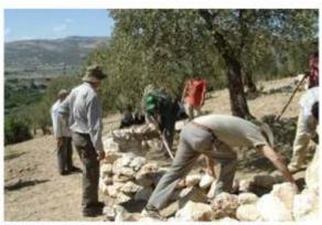
Science plus self-help: the community in Afrin builds simple stone structures to reduce water runoff and soil erosion.
